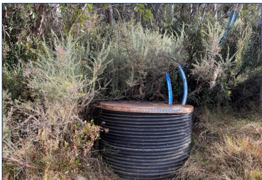
Figure 6 | Example steel pit for a lance type snow gun to be removed (Source: Applicant's Documentation)
