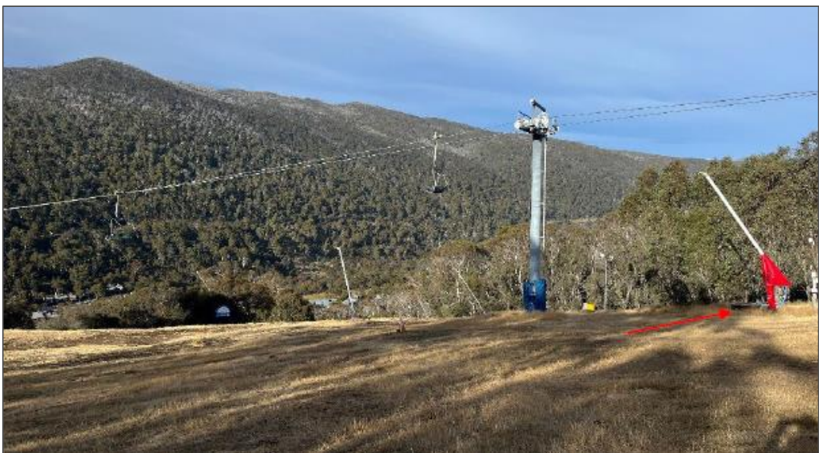
Figure 12 | An existing pit and lance gun to be replaced with new fan pit, TT10 fan gun and lateral from snowmaking mains on the '100 line'. (Source: Applicant's Documentation)
